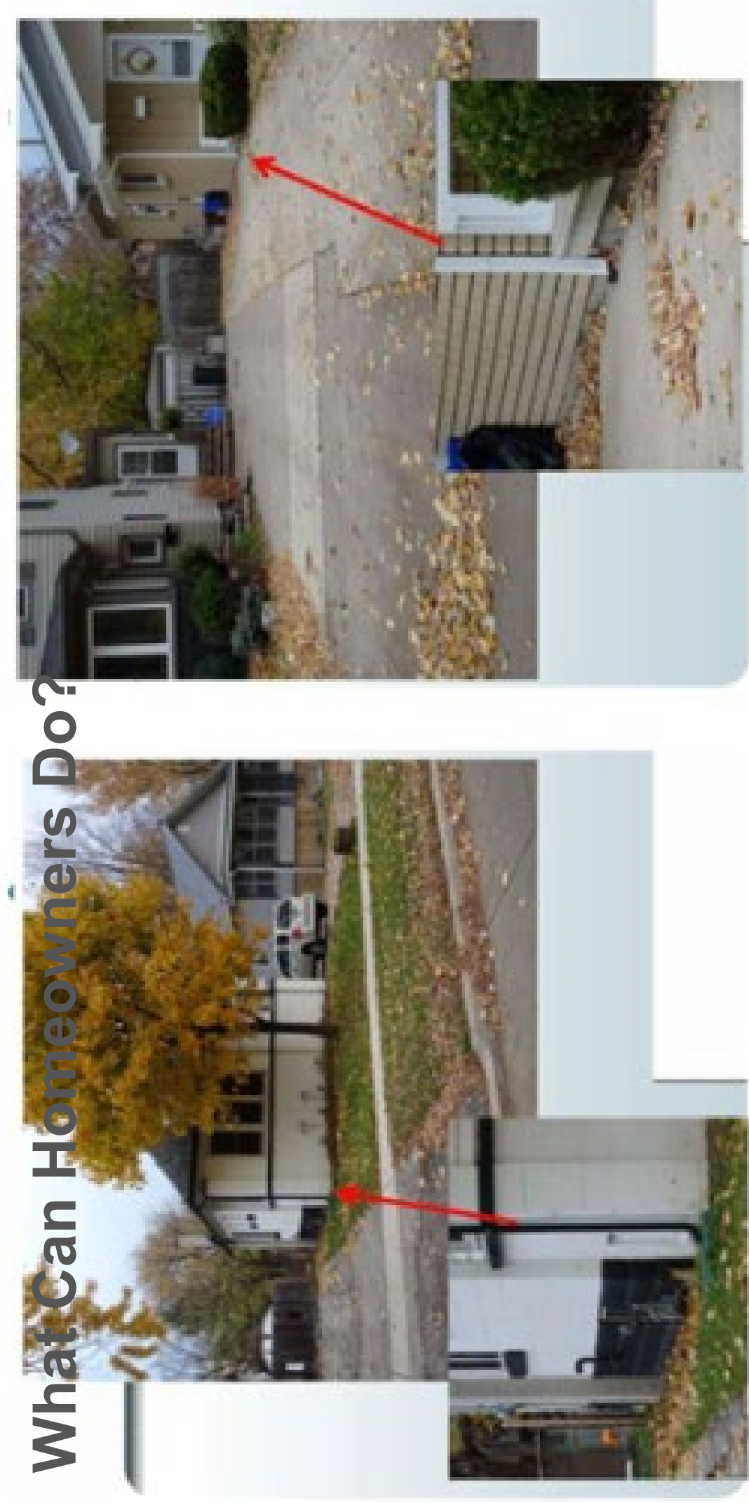
Disconnected Downspout
